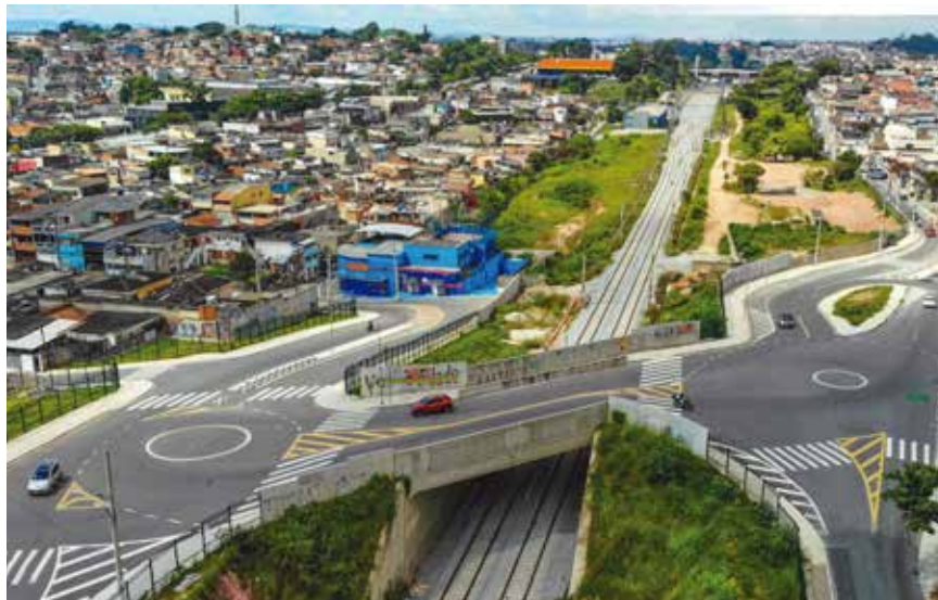
Micronesia Highway Viaduct
