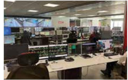
Barcelona Operation Control Center
