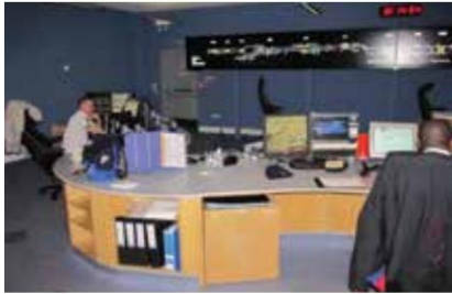
London Underground CCO with Monitoring Ongoing (2013)
